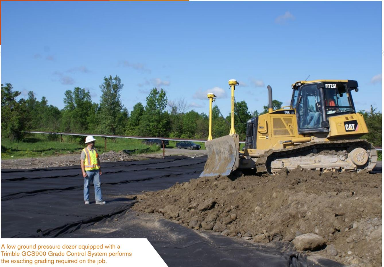
A low ground pressure dozer equipped with a Trimble GCS900 Grade Control System performs the exacting grading required on the job.
