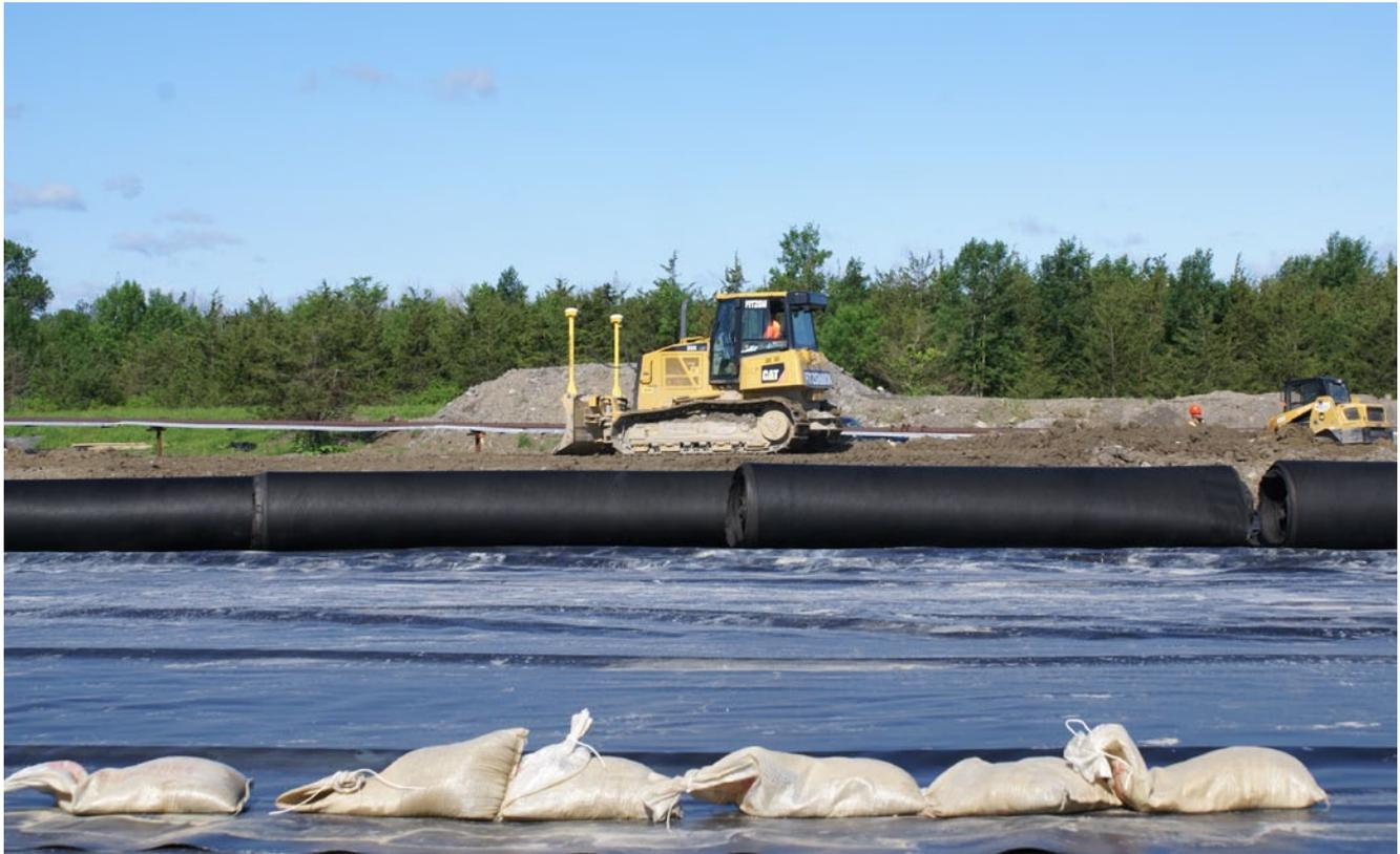
The dozer with the Trimble GCS900 was used to ensure that the amount of fill used in each capping layer is accurate.
